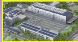
Kasai Plant in Hyogo Prefecture (SANYO Electric)
