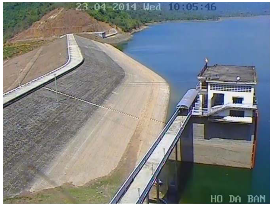
Image from surveillance camera at spillway in Da Ban reservoir, Southern Vietnam
