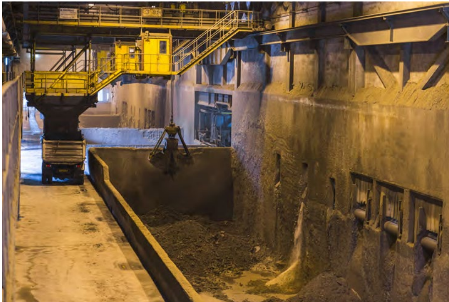
Ash pit at Tuas South Incineration Plant
