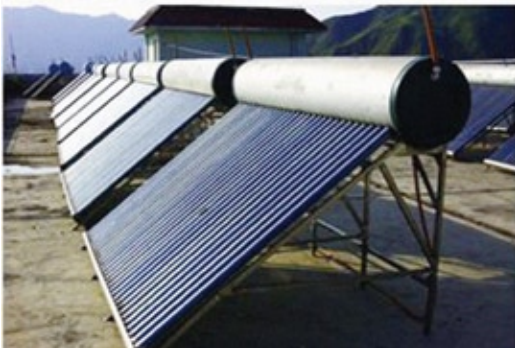
Roof Solar Water Heater
