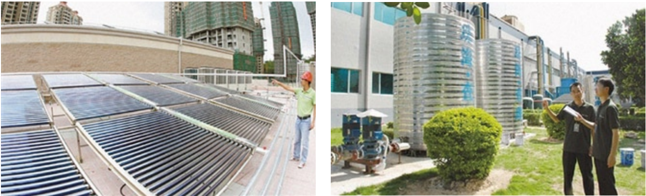
Chart 3-25: New Building's Solar Water Heater System and Geothermal Heat Pump System in Zhuhai
