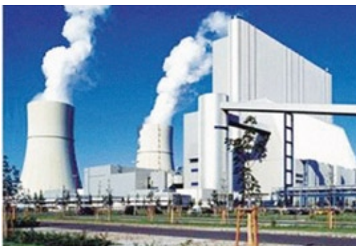
Shanghai Shidongkou Power Plant
