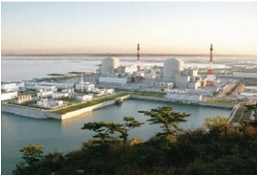
Tianwan Nuclear Station
