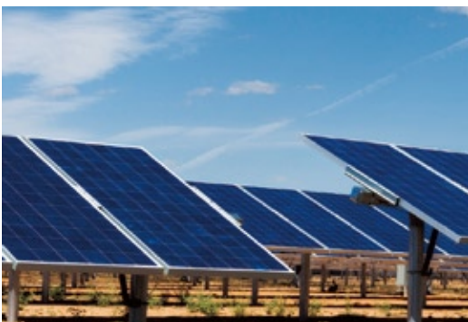
PV Station in Yunnan
