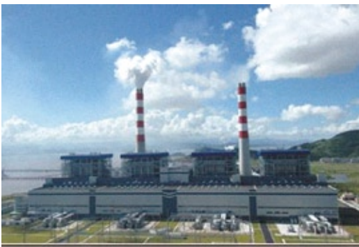
Yuhuan Ultra Supercritical Coal-fired Units
