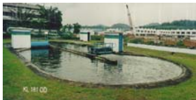
Oxidation Ditch
