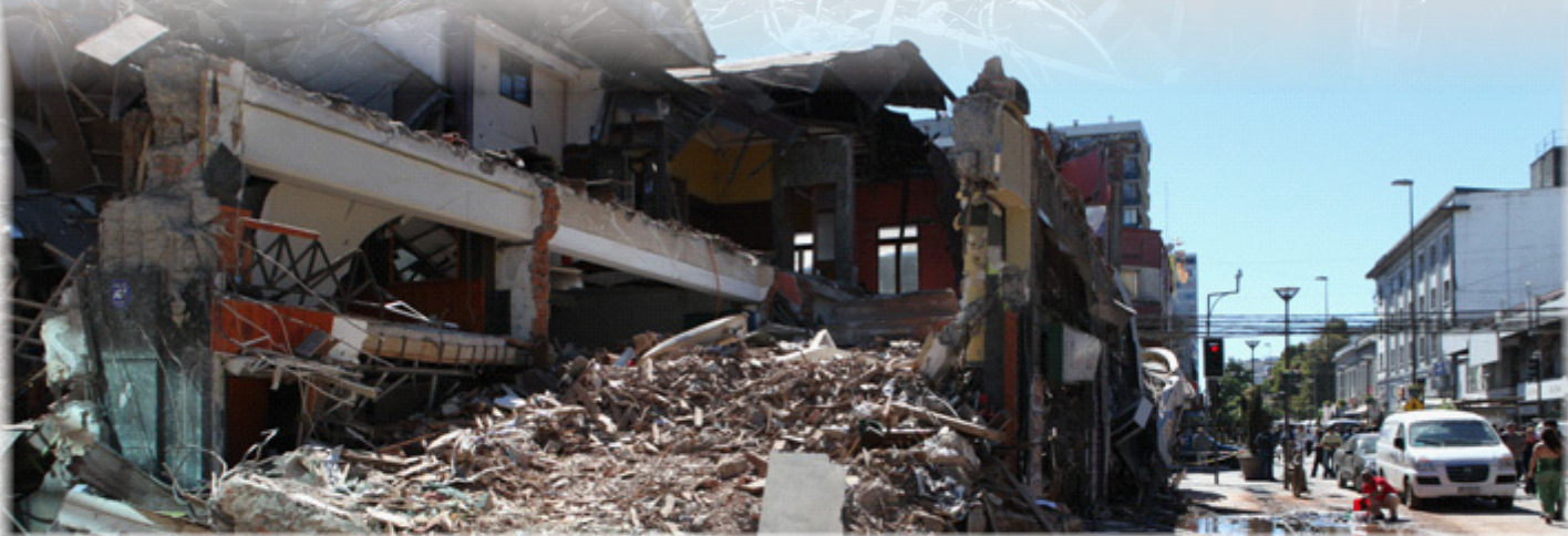
Damage to structures in downtown Concepcion, Chile, due to the February 27, 2010, earthquake. Photograph courtesy of Walter Mooney, USGS.
