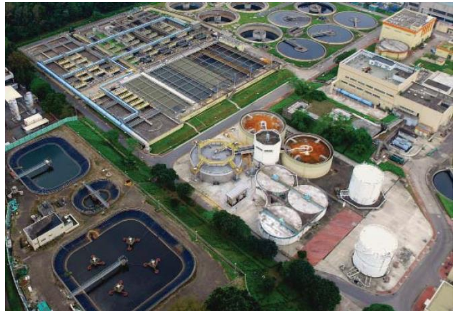
Tai Po Sewage Treatment Works trials co-digestion
