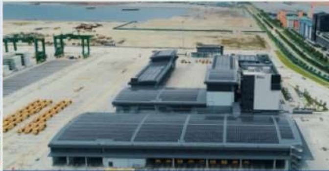
Solar Photovoltaic Panels
