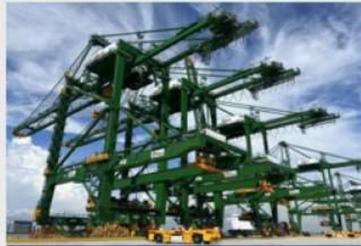
Electrified Quay Cranes
